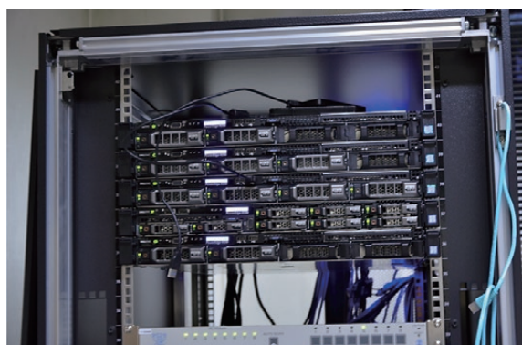
演習室用サーバ Servers for Seminar Rooms
